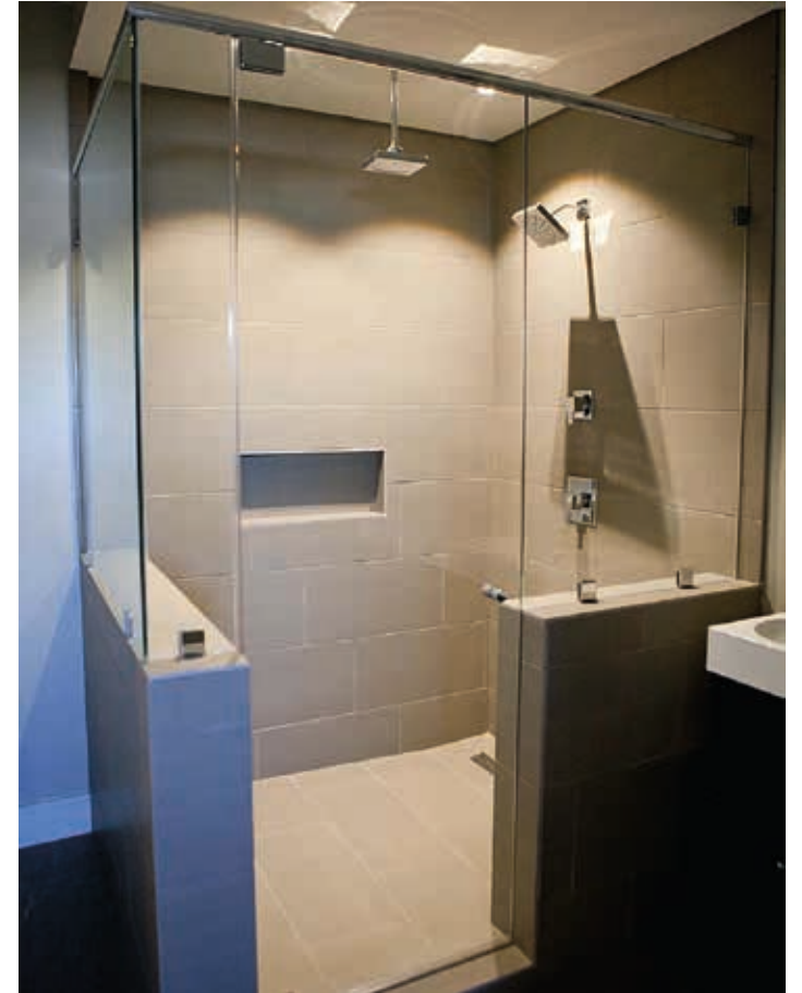
C. Bennett installs premium glass shower doors that are uniquely customized for each home.
