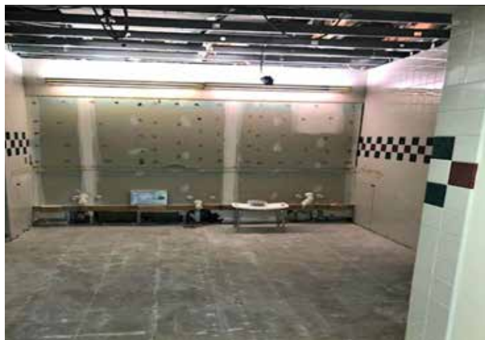
(Men's Restroom Demolition - In progress)
