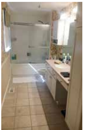
Before Bathroom Remodel.
