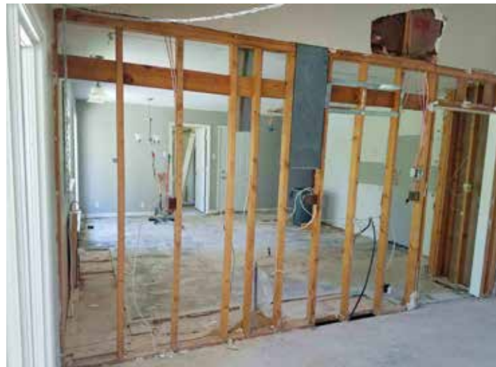
Kitchen wall to be removed.
