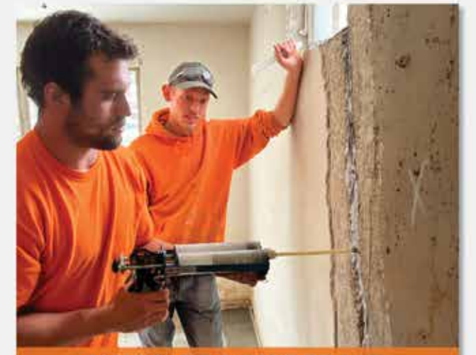
WALL CRACK REPAIR
