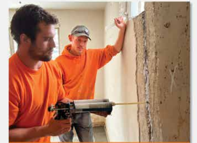
WALL CRACK REPAIR
