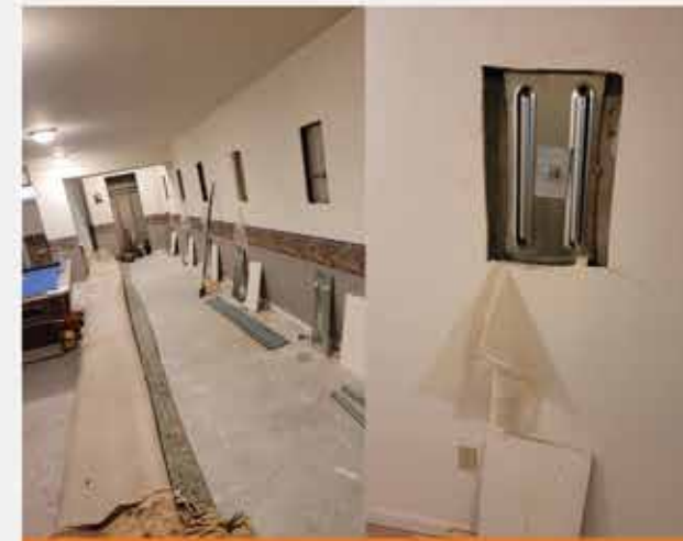
BOWED WALL REPAIR
