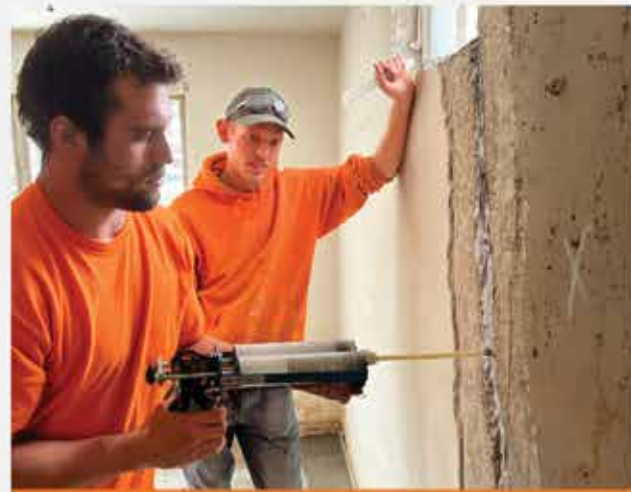
WALL CRACK REPAIR
