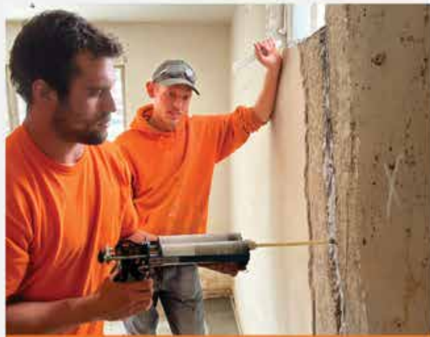
WALL CRACK REPAIR
