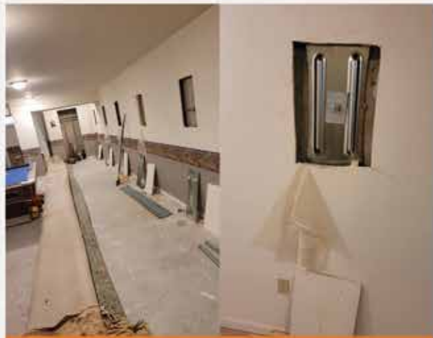
BOWED WALL REPAIR
