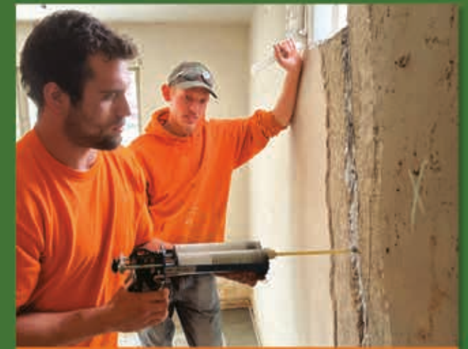
WALL CRACK REPAIR
