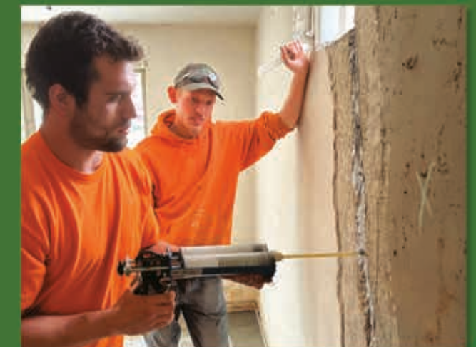
WALL CRACK REPAIR
