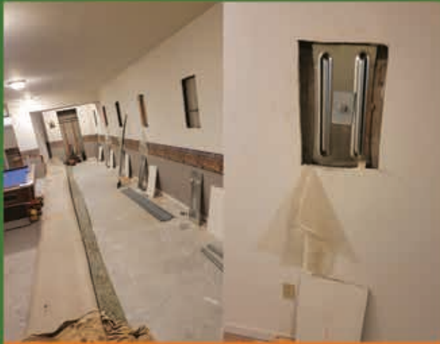
BOWED WALL REPAIR
