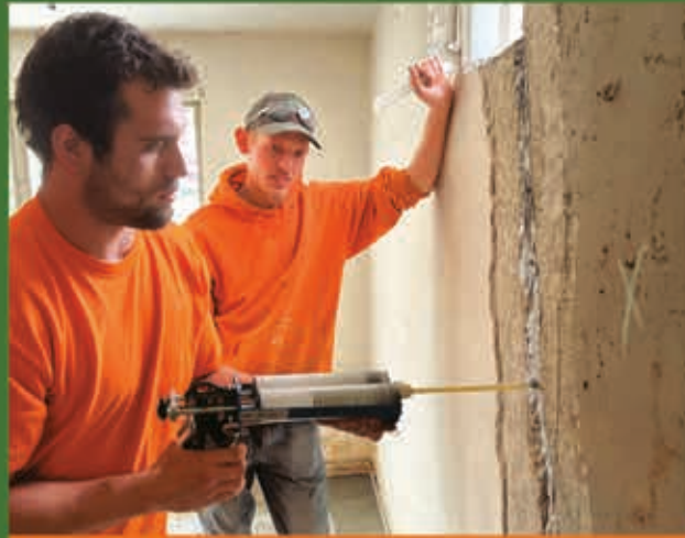
WALL CRACK REPAIR
