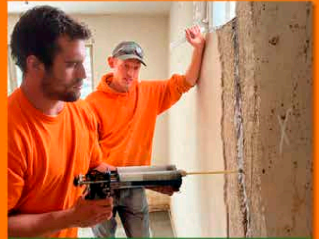
WALL CRACK REPAIR
